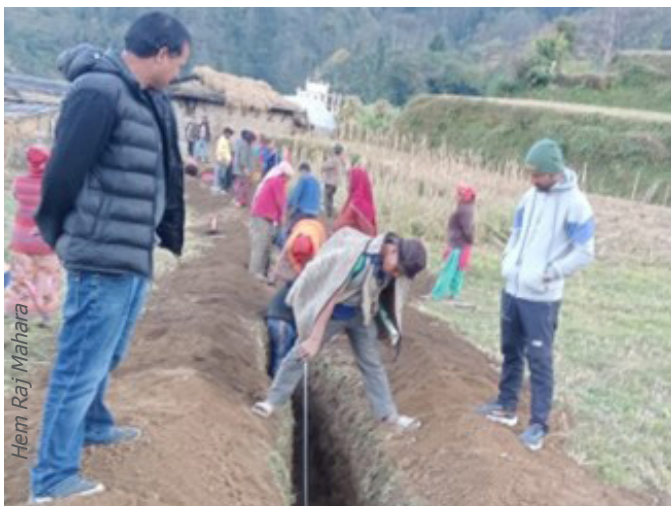
Excitement brought by the project: Local community engaged in digging pipelines
