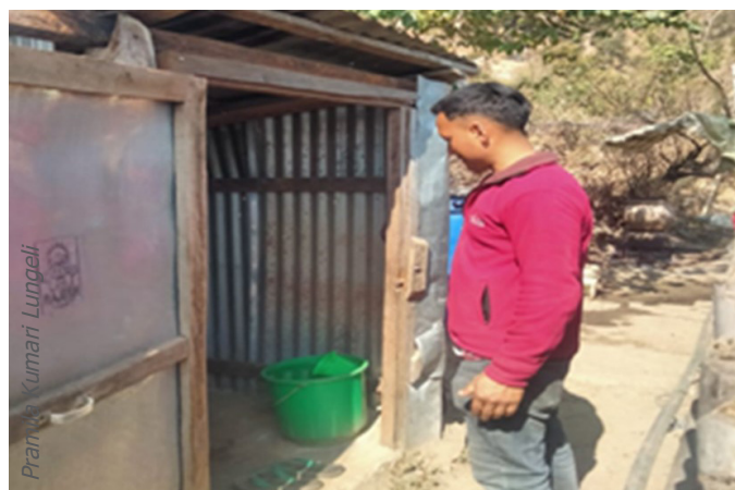
A Volunteer team member inspecting WASH structures
