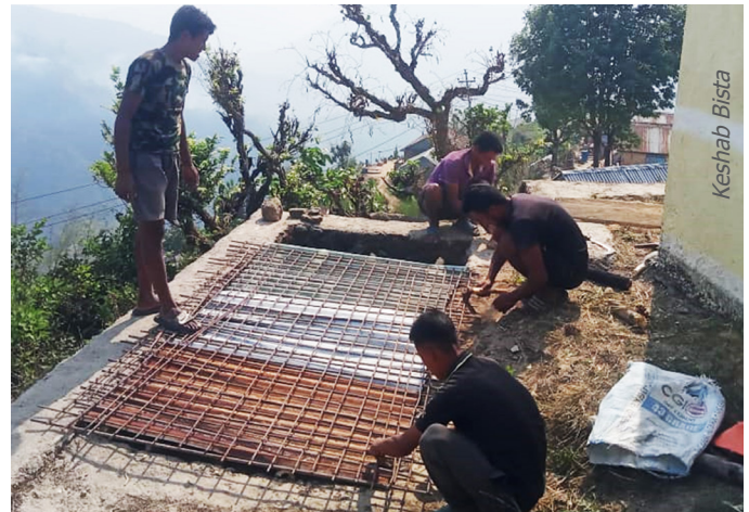
Constructing the slab for the septic tank of the school toilet
